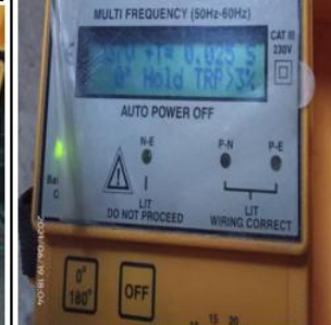
04. Basement area Chiller room
