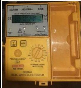
01. Main Panel Area
